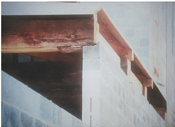
Figure 2. Joisted Masonry Construction
