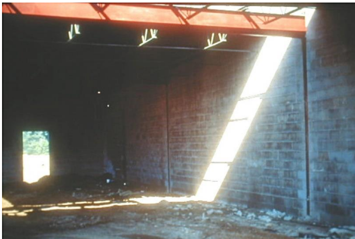
Figure 4. Masonry Non-Combustible Construction
